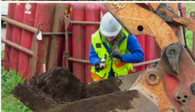
Excavation crew working in Unalaska
